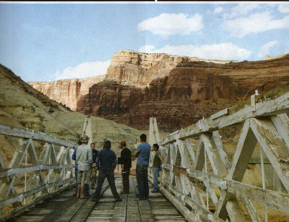
Taking a stroll along the San Rafael Suspension Bridge – built 1935-37 – the last one of its kind still standing and listed on the US National Register of Historic Places
